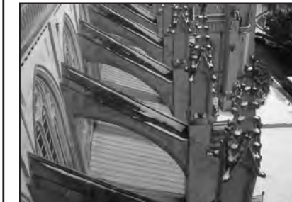
Flying buttresses add support to the walls of the Washington (D.C.) National Cathedral.
