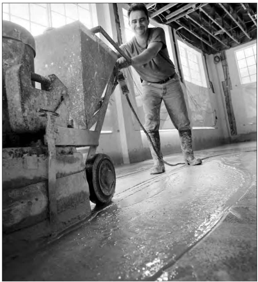
Steve Toffoli does a rough grinding to expose newly installed terrazzo floors at the Betsy Ross Hotel in South Beach, Fla., recently. by his grandfather, Louis Toffoli. "It's in my blood," said Toffoli, 39, of Doral, Fla.-based Creative Terrazzo.
