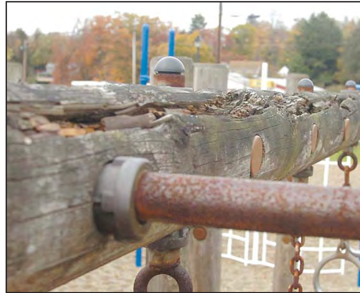
A rotting piece of wood supports a set of rings that children cross.
